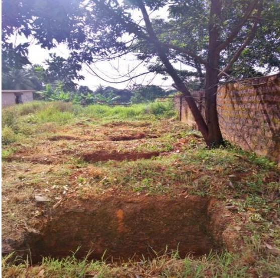
RAIN WATER HARVESTING PITS
